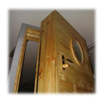
It is accepted practice to build very well insulated walls and roofs (for example with 40cm of straw, or 35cm polystyrene) with U wall less than 0.15 or 0.1, but it seems to us deplorable not to have doors insulated to the same level. Using two doors takes up valuable space and only slightly reduces the energy loss.
